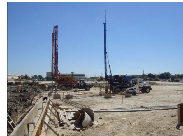
Piers being drilled for the foundation of the Data Center.
